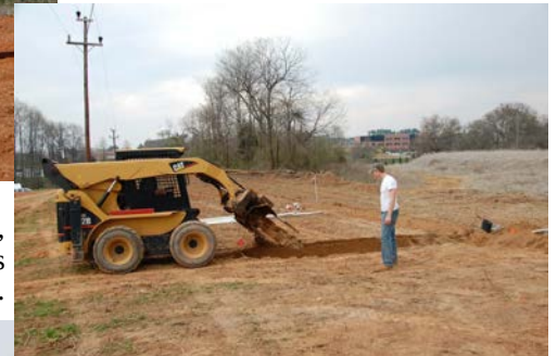
David Settle in the Bobcat, and helper, prepare the ground and lay the trenches for the water lines for the nursery.
