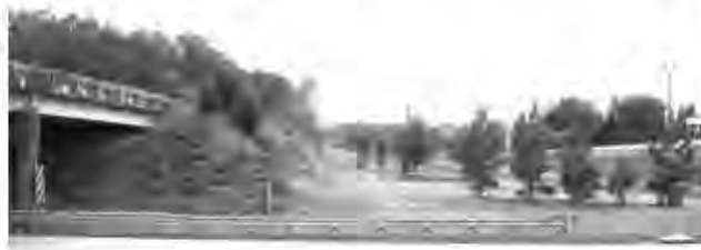
The Interchange at US-221 and SC-295 looks good.
