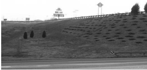
The Interchange at I-26 had problems from the beginning, but Club work is improving it in 2010.
